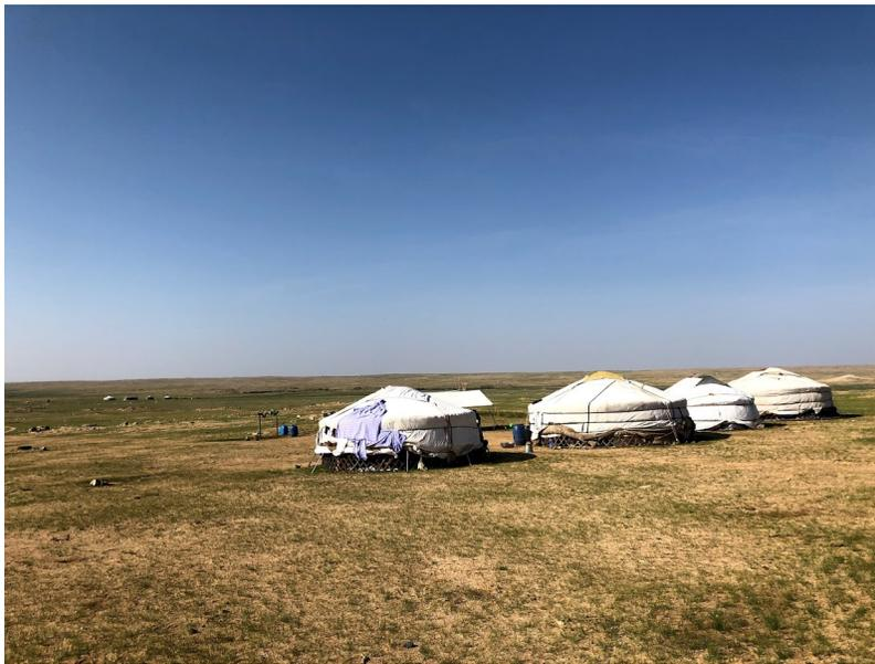
Figure 1: Four gers (Mongolian yurts) in Mongolia's Sukhbaatar Province, with several more gers in the distance on the left. On warm days, the insulating felt of the ger may be rolled up to create greater air circulation, as shown in the photo above. Credit: Jake Kalodner, permission granted.
